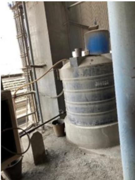
The addition of grinding aid chemical to cement clinker is operated in a closed PID loop, before it reaches the mill for crushing. The chemical dispensing depends on clinker weight on the conveyer belt. More the clinker, more the RPM of dispensing pump is increased to add more chemical.
